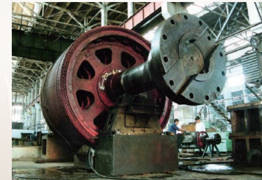
urgent repair of large motor
