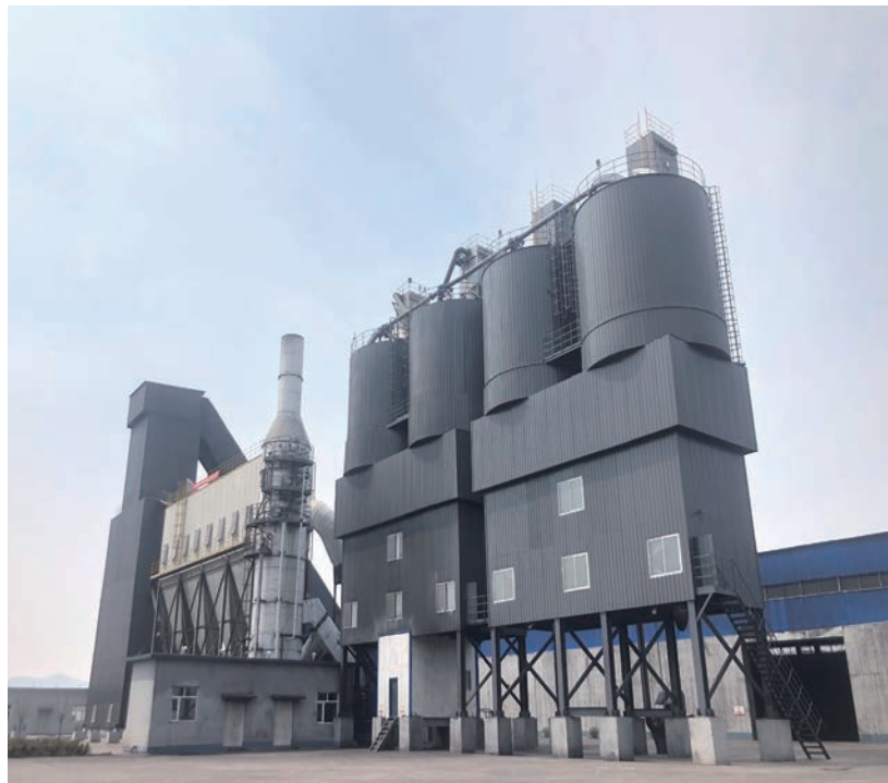
Lingyuan pulverizing coal EPC project
