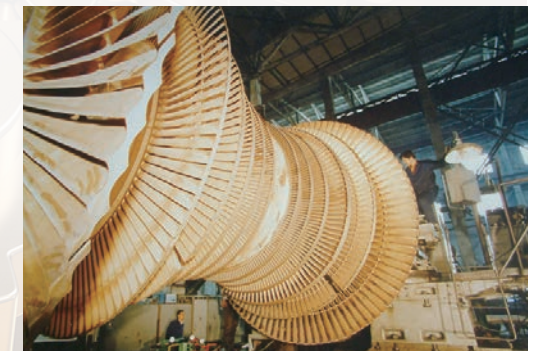
urgent repair of 320MW turbine rotor
