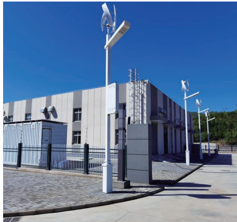
State Grid Zhangjiakou Chongli 10kV multi-energy complementarity demonstration project
