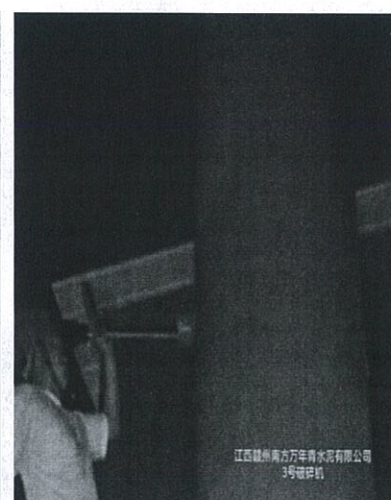
锤式破碎机废气排放口#3
