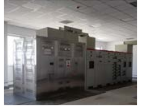
10KV/6KV/5000KVA Transformer
