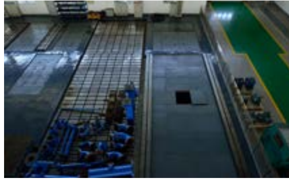
Open Pump Test Loop- Installation Platform & Water Pool
