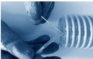
Step 5: Separate the grounding wire and hose wall by carefully pulling them apart. Cut off the loose end of the hose wall with the side-cutter.
